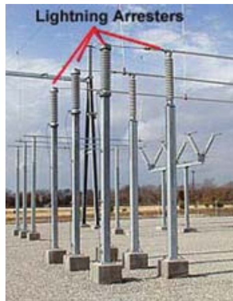
Lightning arresters on bus structures
